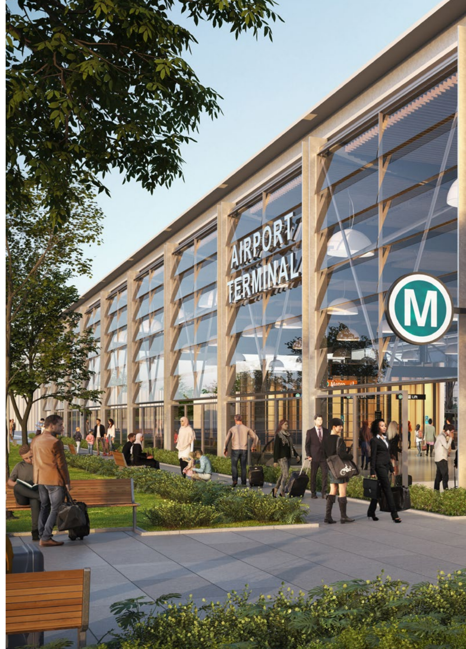
An artist's impression of the Airport Terminal Station – Sydney Metro Western Sydney Airport.
