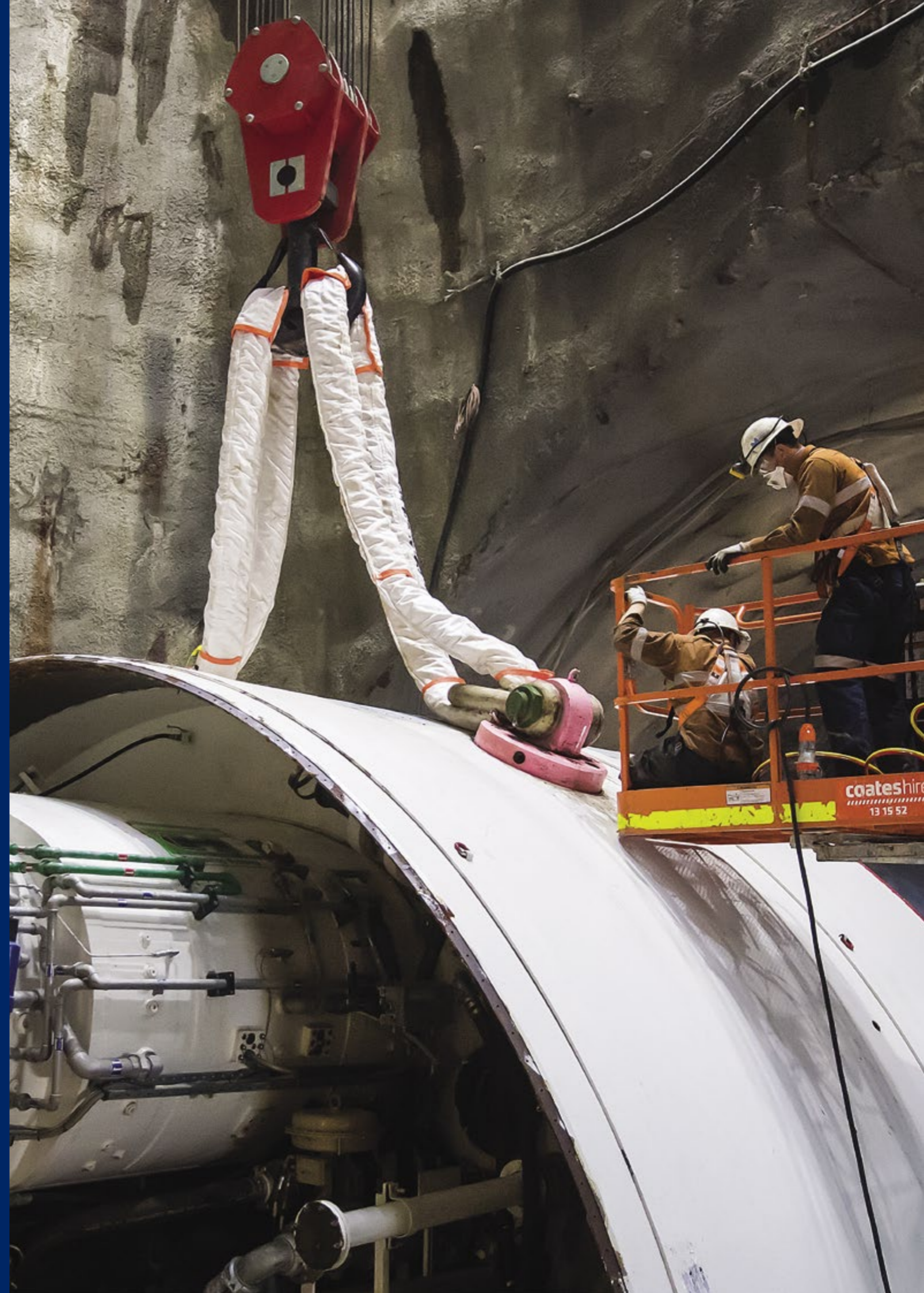
A TBM being assembled on the Sydney Metro City & Southwest project.
