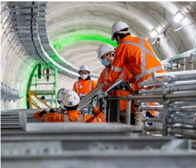
A safety walkway is installed inside the Sydney Metro tunnels.
