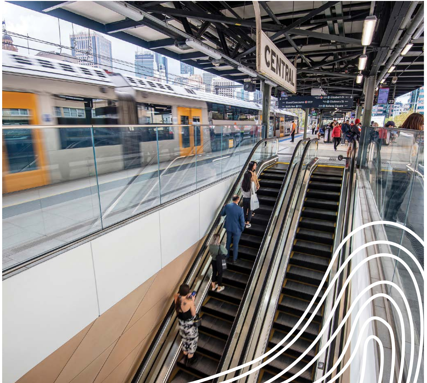
In preparation for Metro services at Central Station escalators have been installed to provide convenient access to suburban platforms.
