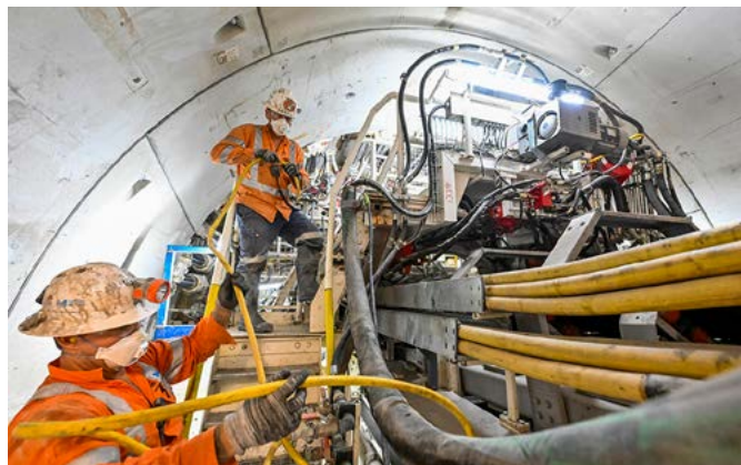
Installation of tunnel segments.
