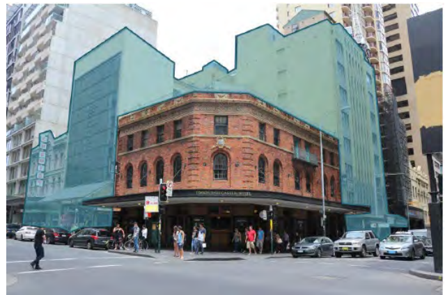
Picture 17 View prior to building demolition (2016)
