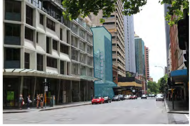
Picture 20 View prior to building demolition (2016)
