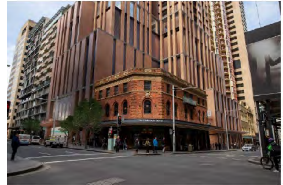
Figure 40 – Artist's impression of south station podium viewed from north west at Pitt Street / Bathurst Street intersection (source: Arterra Interactive)
