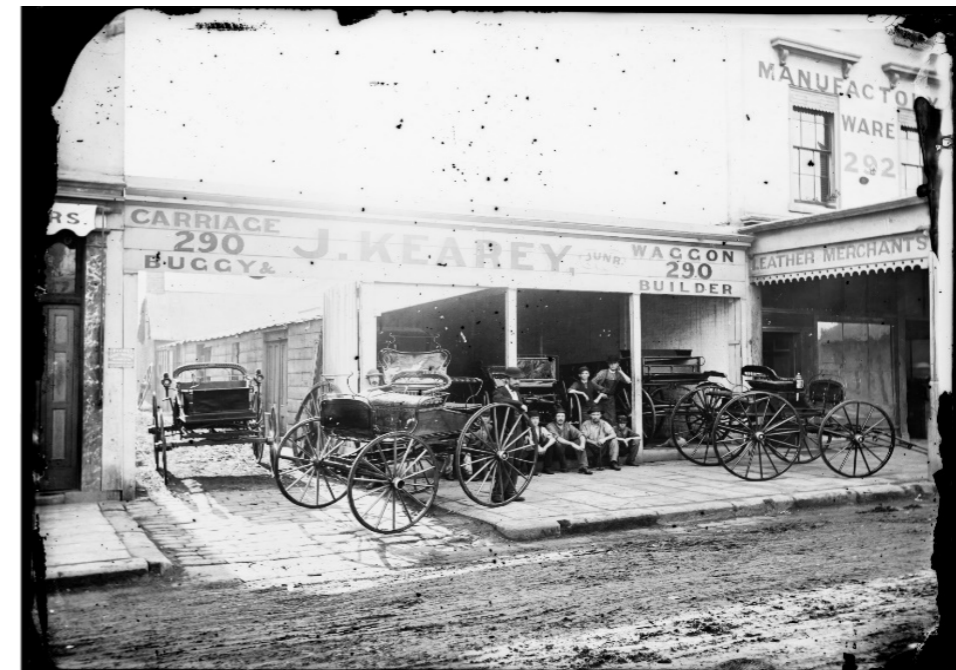
Figure 44 – A buggy manufacturer on the OSD north site
