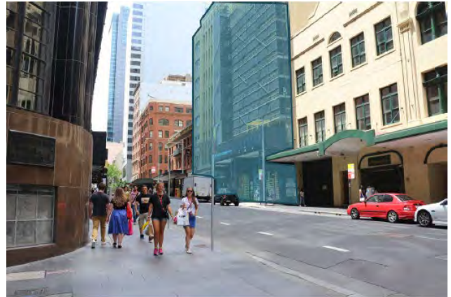
Picture 26 View prior to building demolition (2016)
