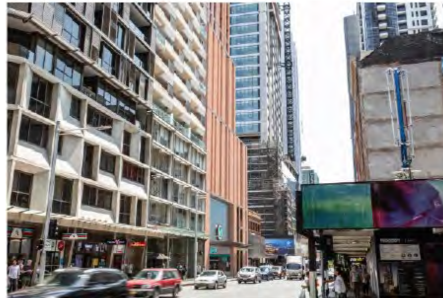
Figure 39 – Artist's impression of south station podium viewed from east along Bathurst Street (source: Unsigned Studio)
