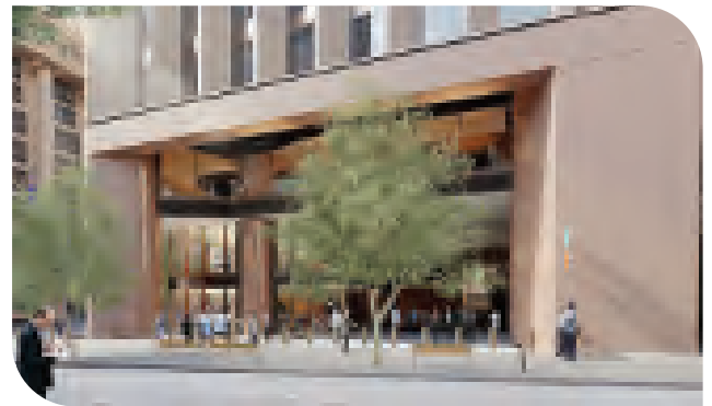
West elevation of the podium viewed from Castlereagh Street.
