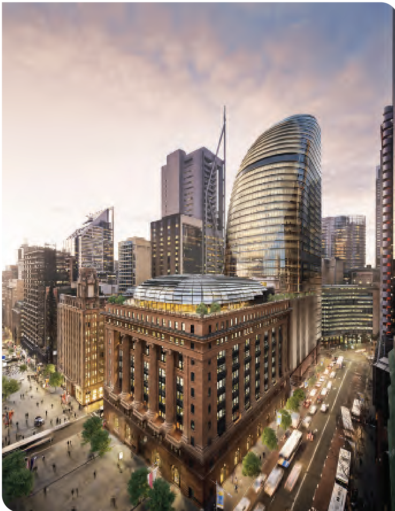
The southern elevation of the North Tower façade viewed from Martin Place showing its relationship to the podium below and the relationship of the 'southern lens' to the 50 Martin Place glazed roof dome.
