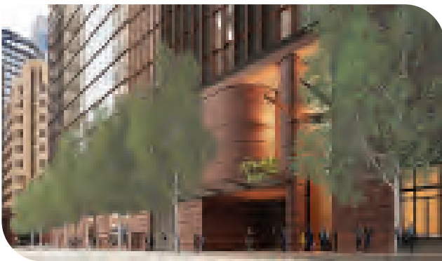
Podium viewed from Castlereagh Street with commercial lobby entrance in the foreground and retail strip in the background.
