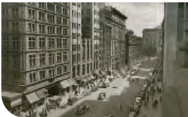
Historical photo of Martin Place, 1959. Source: NSW State Archives
