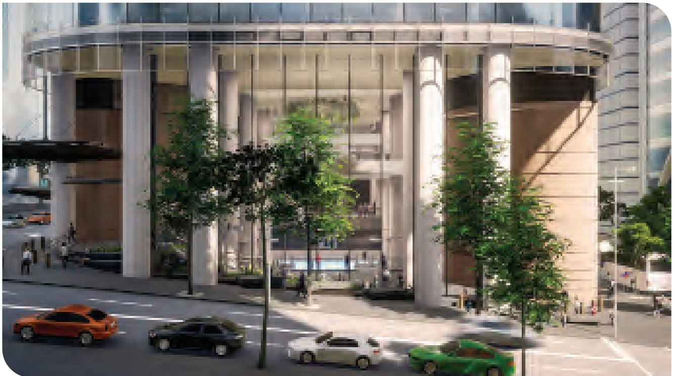
North elevation of the podium viewed from Hunter Street with station entrances at the corners. The glazed façade reveals the entrance hall and internal soft landscaping beyond, with crafted stone elements outside that act as hostile vehicle mitigation devices along this façade.
