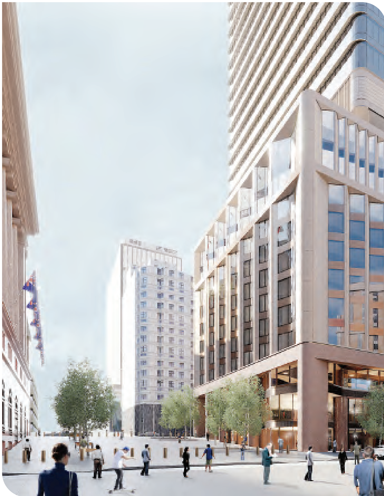
View of Martin Place plaza fronting the south integrated station development.
