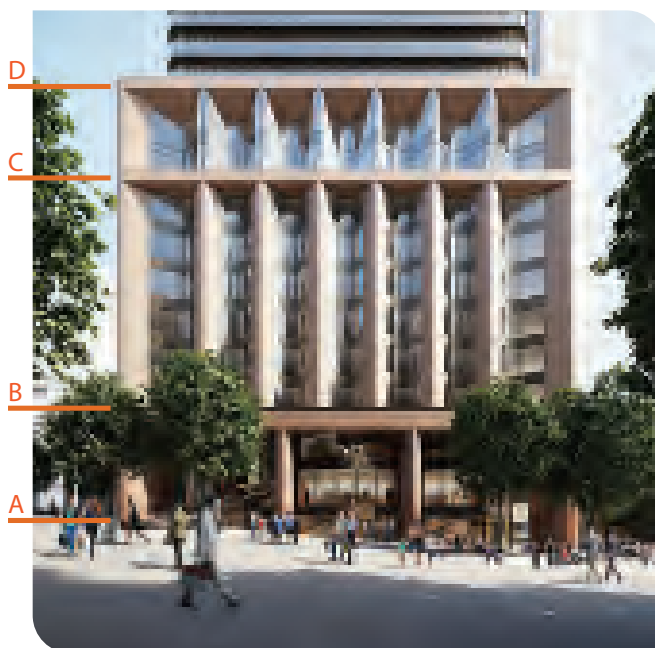
South Tower podium viewed from Martin Place with delineation of podium zones identified
