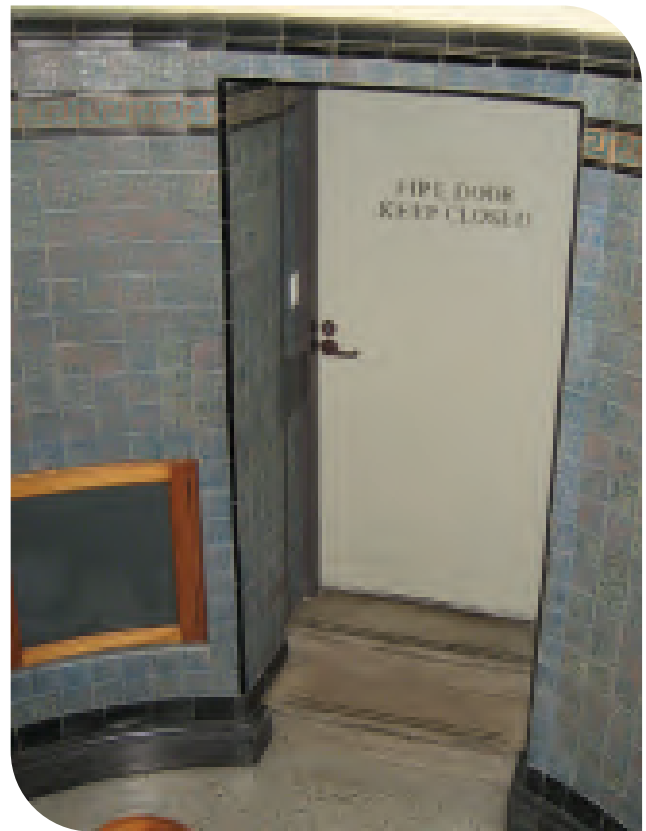
Stairwell with 1960s openings.
