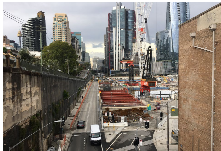
Figure 3.7 Heritage wall along Hickson Road, 2021 Source: Arcadia Landscape Architecture
