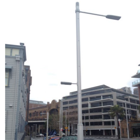
Figure 4.33 Smart Pole - Walsh Bay Source: Google
