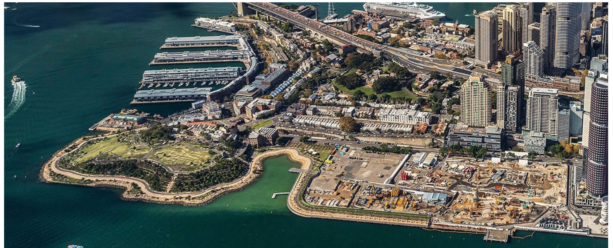
Figure 1.8 Birds view of Barangaroo https://www.barangaroo.com/the-project/infrastructure-nsw/
