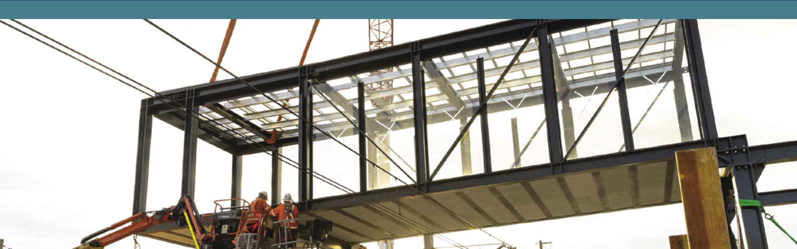
Installation of the new pedestrian concourse at Dulwich Hill Station.
