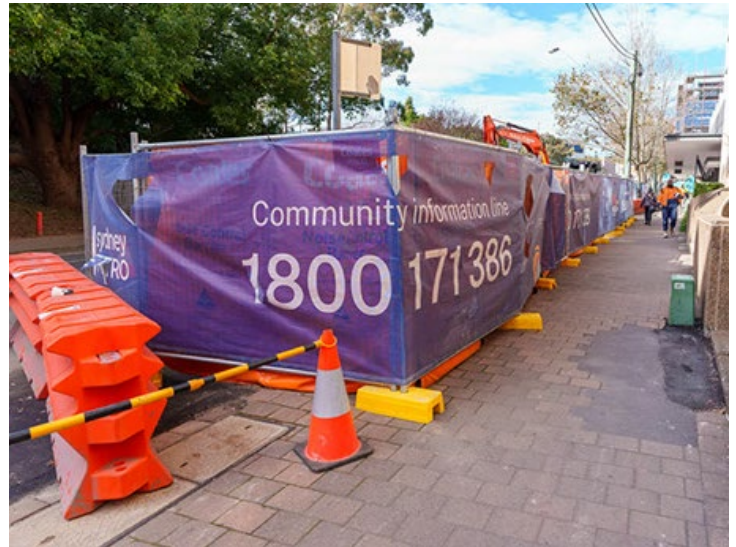
Image of noise blankets around equipment
