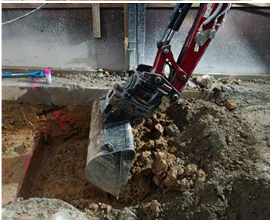
Images of excavators being used for work activities.
