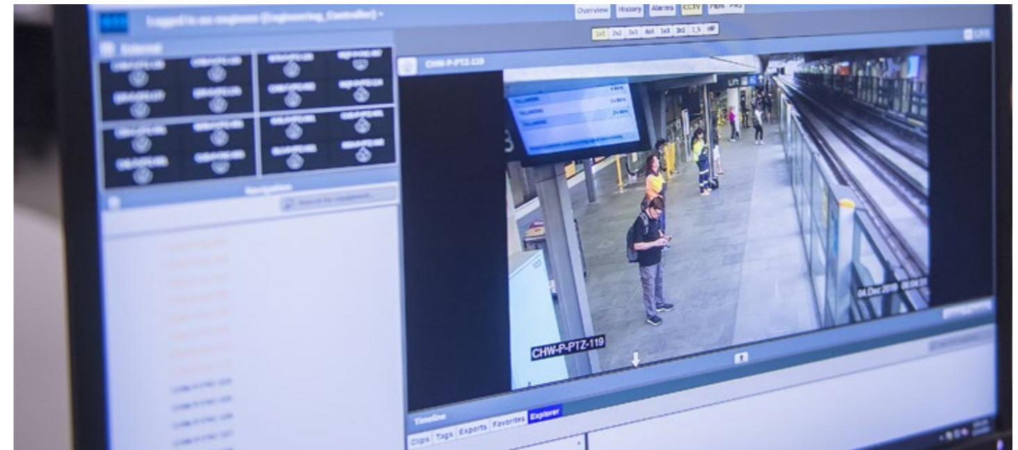
Expert train controllers work in a state-of-the-art Operations Control Centre at Tallawong.
