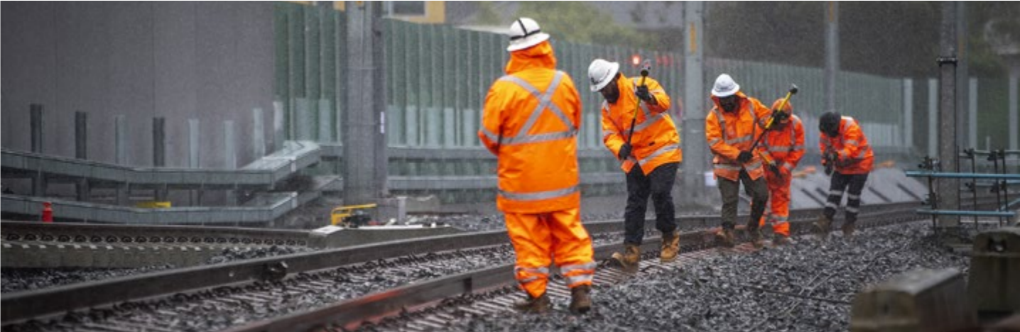
Track cutting works between Artarmon and Chatswood stations.
