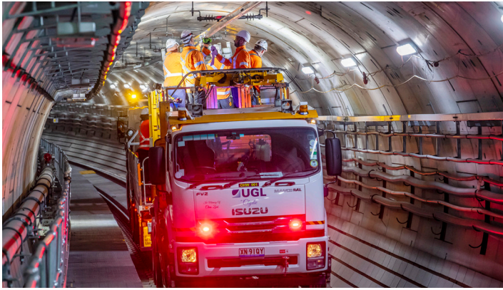
The overhead wire being installed in the tunnels beneath Sydney Harbour.
