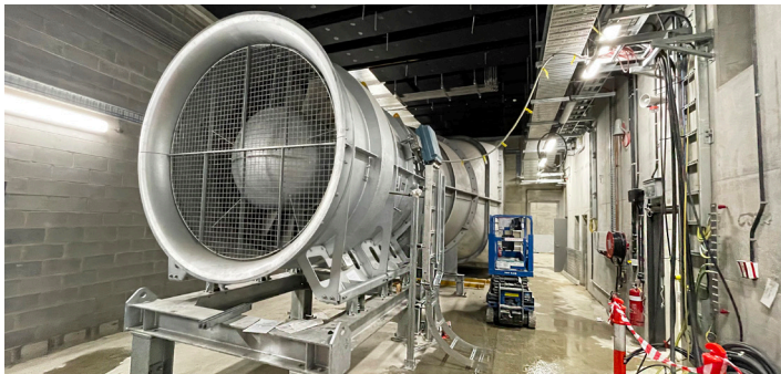
One of the giant ventilation fans being installed above the twin tunnels.
