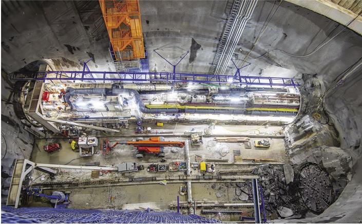
TBM Peggy breaking through at the Airport Terminal temporary shaft while TBM Eileen is traversing the shaft.
