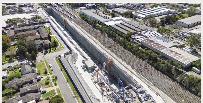
The incredible 12-month transformation at St Marys, with the station box now fully excavated and lined with concrete.
