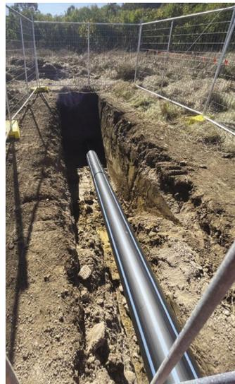
Pipe installed via horizontal directional drilling method across Mamre Road.
